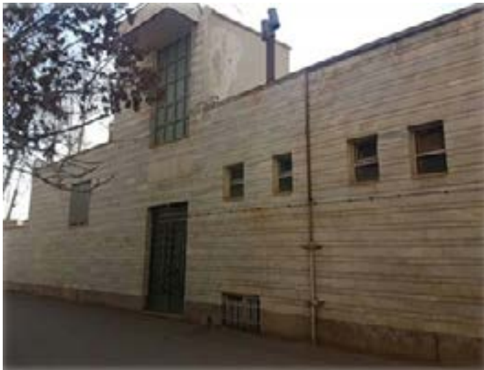
Figure 1. Real building in Isfahan city.
